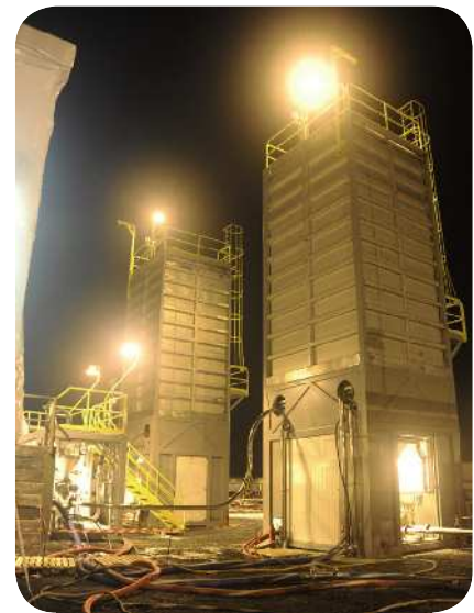
Carbonate and Polymer Skid Mounted Silos
